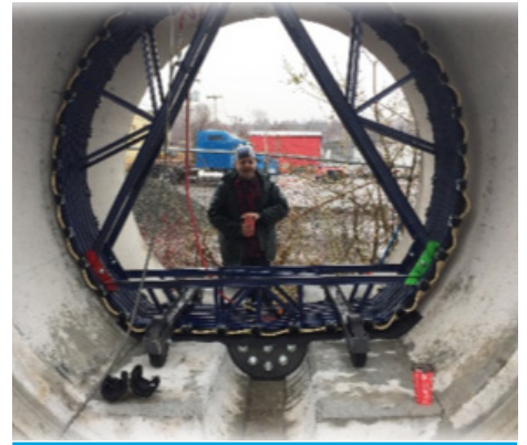
Packer for pipe 96" pipe with cunette
