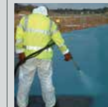
Bridge deck Waterproofing
